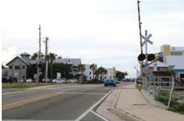
In 2015, MDOT added lights and gates to this intersection in Bay St. Louis. (Photo special to The Pelahatchie News)
