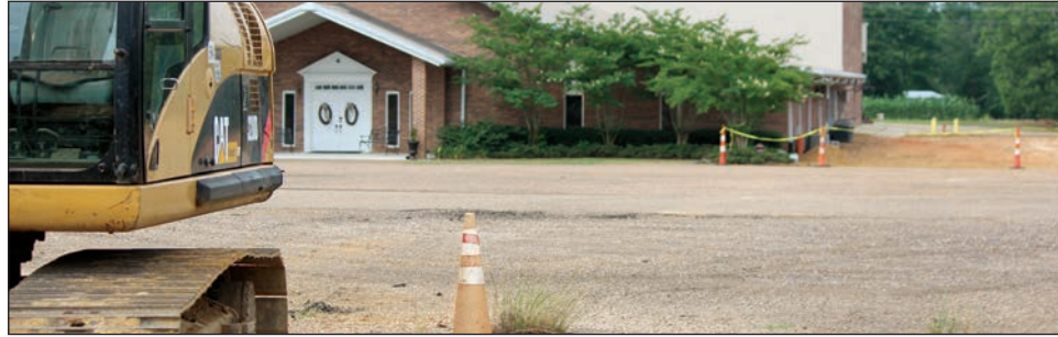
Construction to Cross Roads Baptist's parking lot (Photo special to The Pelahatchie News)
