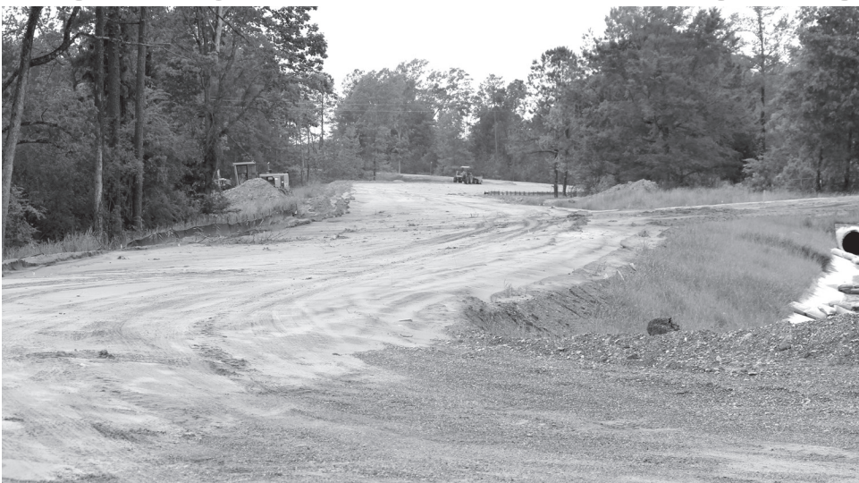
During 2013, the Town of Pelahatchie began working on resurfacing Brooks Avenue to Lake Road, as well as Hwy 80. Other reconstruction efforts include Hwy. 43, where officials are working towards creating a wider and direct passageway through the Cross Roads area of Pelahatchie. (Photo special to The Pelahatchie News)
