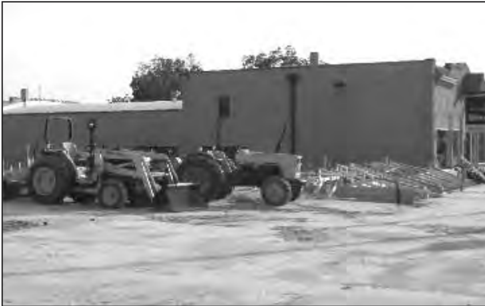
The construction of Brickhouse Fitness Center is well underway. (Photo by: Kristen J. Rials)
