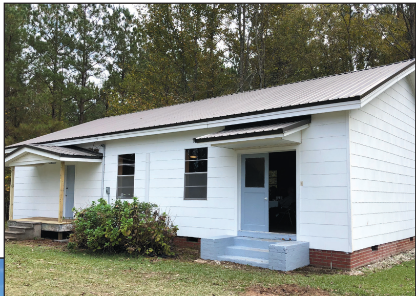
The Rob Fellowship Hall (Photo Above)
